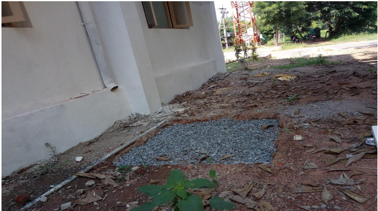
Rain Water Harvesting Pit at F-Block in Campus
