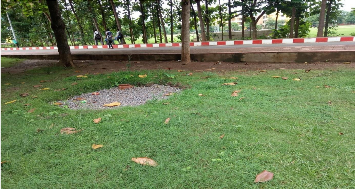
Rain Water Harvesting Pit at A-Block in Campus
