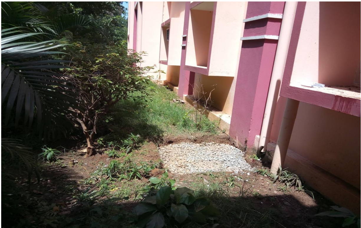
Rain Water Harvesting Pit at D-Block in Campus
