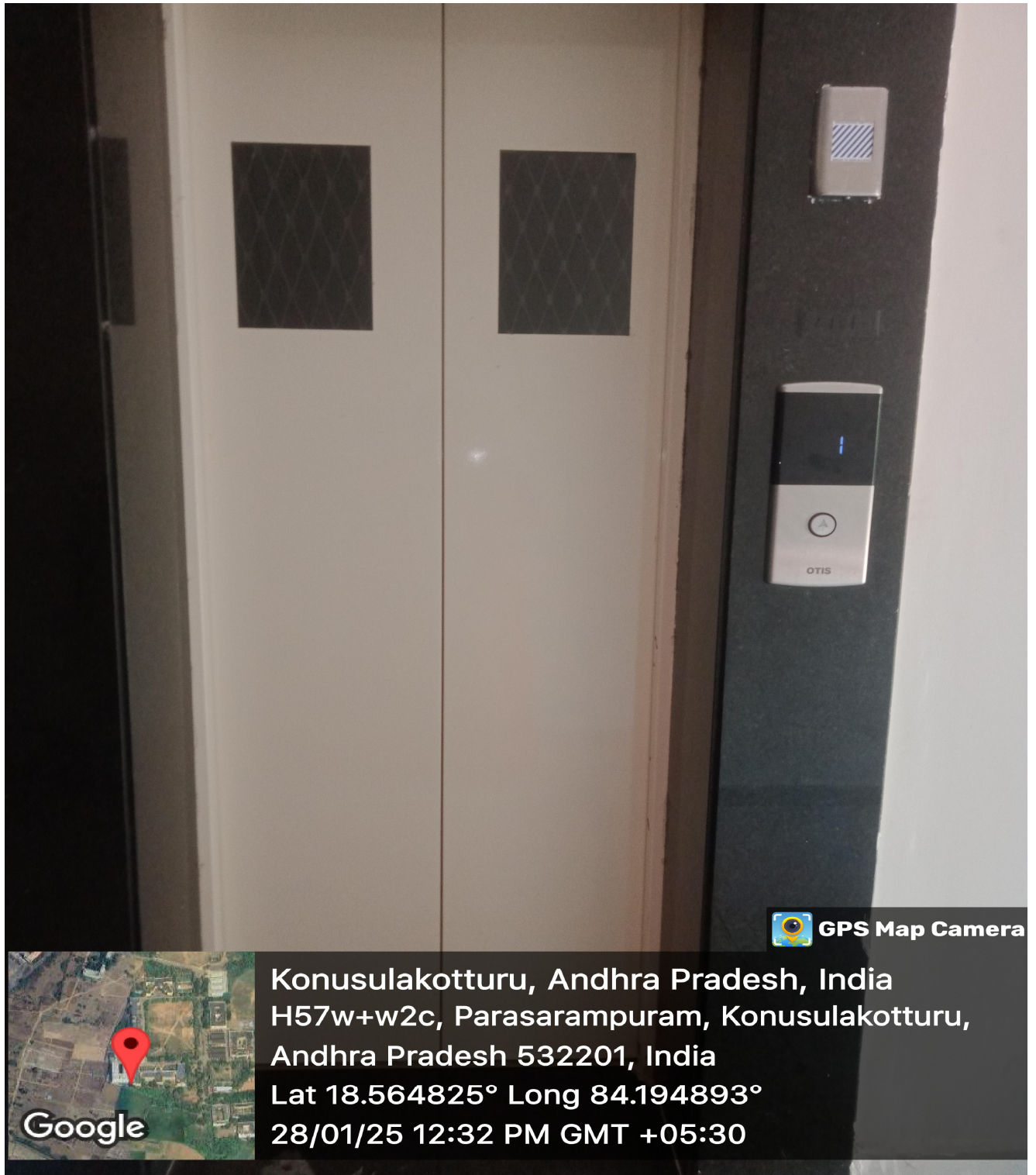
Lift Facility at G Block
