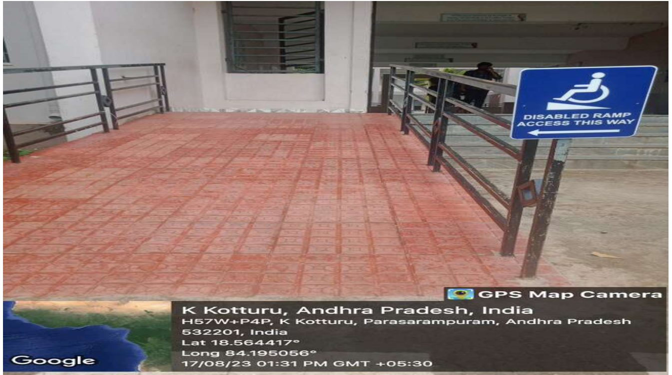
Ramp at E Block
