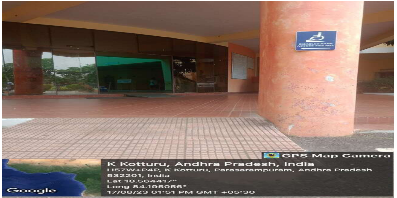
Ramp at C Block
